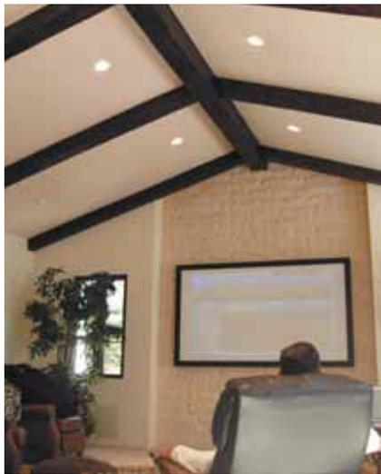
**You can reduce sound reflections by applying a uniform stretched fabric layer to the ceiling, and concealing absorptive and scattering materials behind it.**
